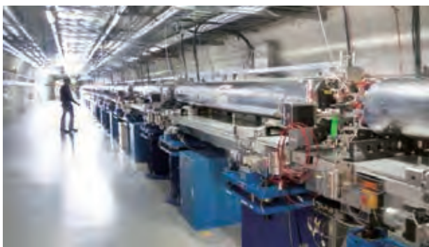
Figure 2. The undulator hall of LCLS, in which the 15 GeV electron beam energy is converted to intense X-ray pulses.
